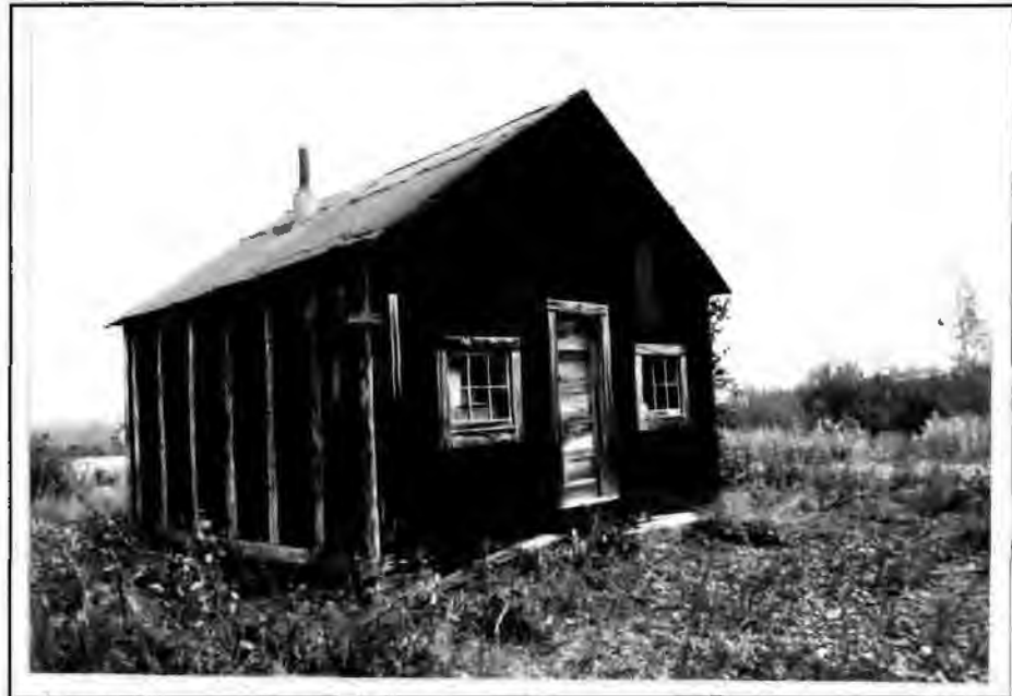
Figure 58. The Byrd/Stevens Garage, 1993. The view is looking northeast.
